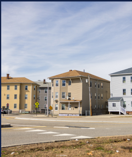
Mill Brook Conduit, a tunnel for water installed in 2007, runs beneath this rotary on Olde Millbury St.
