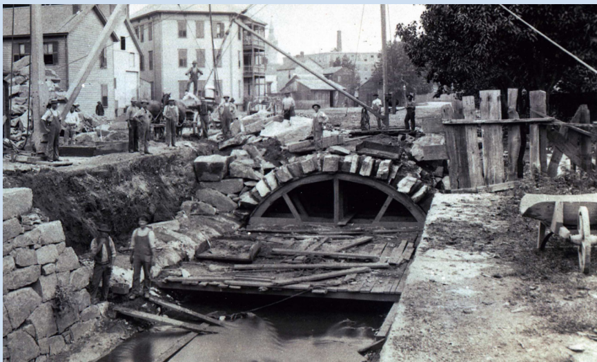
Covering of the Blackstone Canal, C. 1890 | From The Collection Of Worcester Historical Museum
